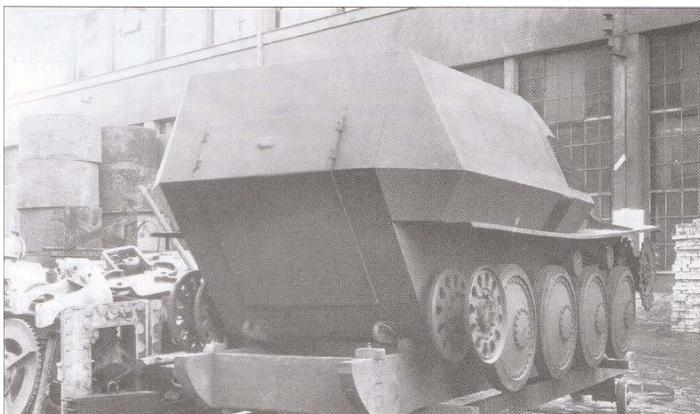
A prototype of the troop carrier, featuring a 38(d) chassis and 251/C body captured by Allied forces after the war. GHQ believes that production models would have utilized the 251/D style doorways.
