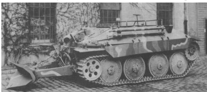
Photograph of prototype 38(d) chassis armoured recovery vehicle.
